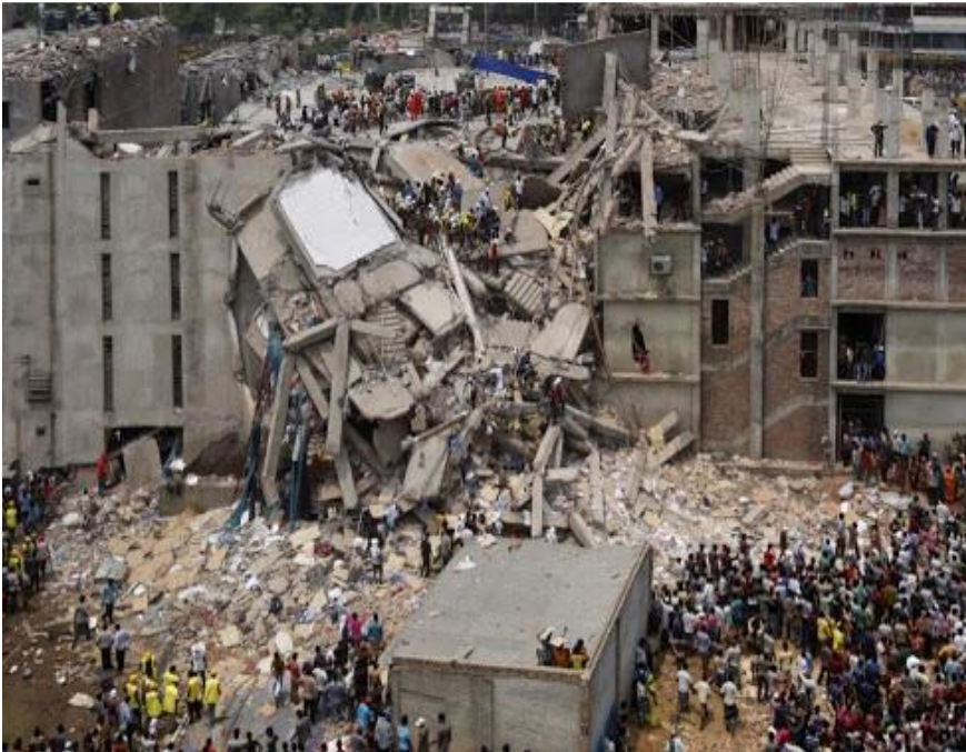
Rana Plaza Collapse, 2013
